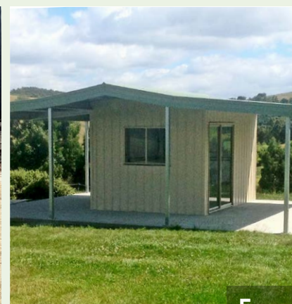
Infrastructure Grant: Constructing intensive care treatment unit.
