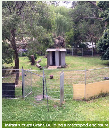
Infrastructure Grant: Building a macropod enclosure.
