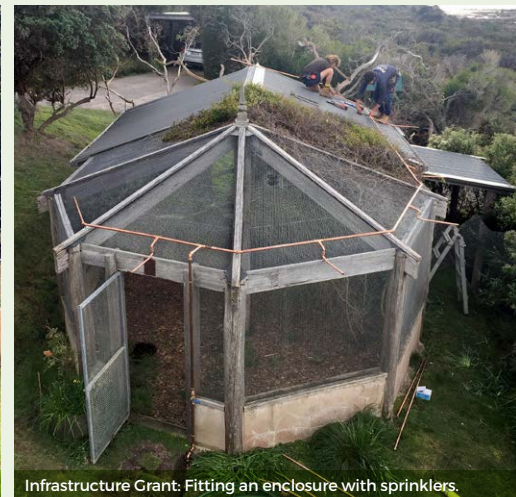
Infrastructure Grant: Fitting an enclosure with sprinklers.
